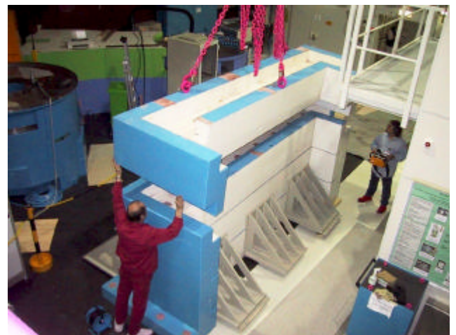
Fig. 4: Assembly of the block house walls
