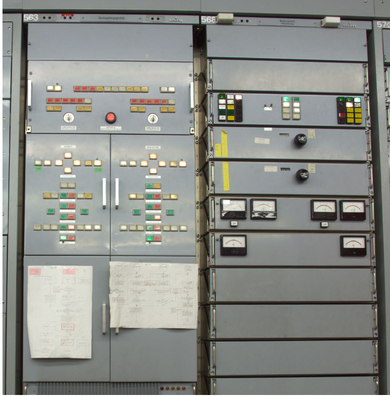
Figure 2.1: The two motion control racks of Raisting 1 . The left rack is the Verriegelungs-gestell , the right rack is the Reglergestell .
