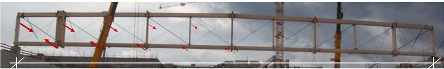
Span  $L = 78$  m, Load  $F = 1100$  tons (60 trucks)
