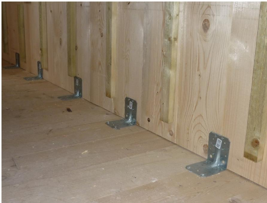
*Fig. 11 Typical CLT wall to slab connection showing ABR105 brackets.*
