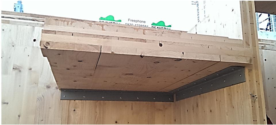
*Fig. 16 Special moment connection for a cantilever stair half landing slab.*
