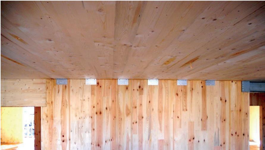
Fig. 3 Floor-to-wall connections at the first storey in a 6 storey CLT building, designed for a medium seismicity area.
