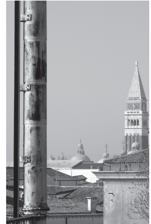
Guide frame of gasholder V with view to the Campanile of St. Mark's Square (Casarin, 2009).
