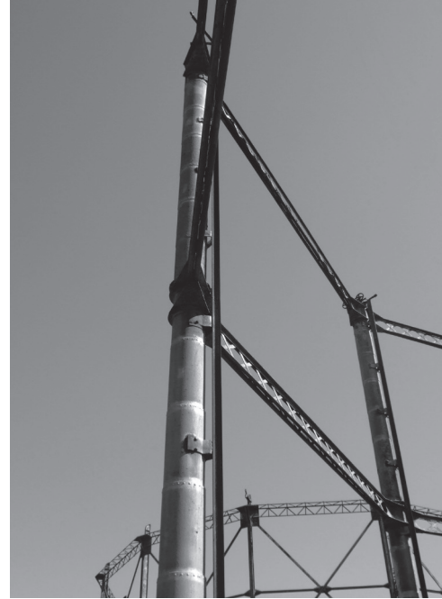
Guide frame of gasholder V (BB 2008).
